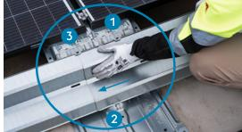
Move the iFIX S deflectors until they reach the end of the row, 40 to 60 mm from the edge of the iFIX S connector.
