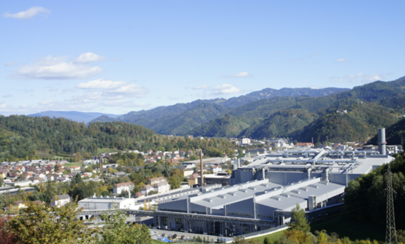
The world's most modern stainless steel plant in Kapfenberg, Austria.
