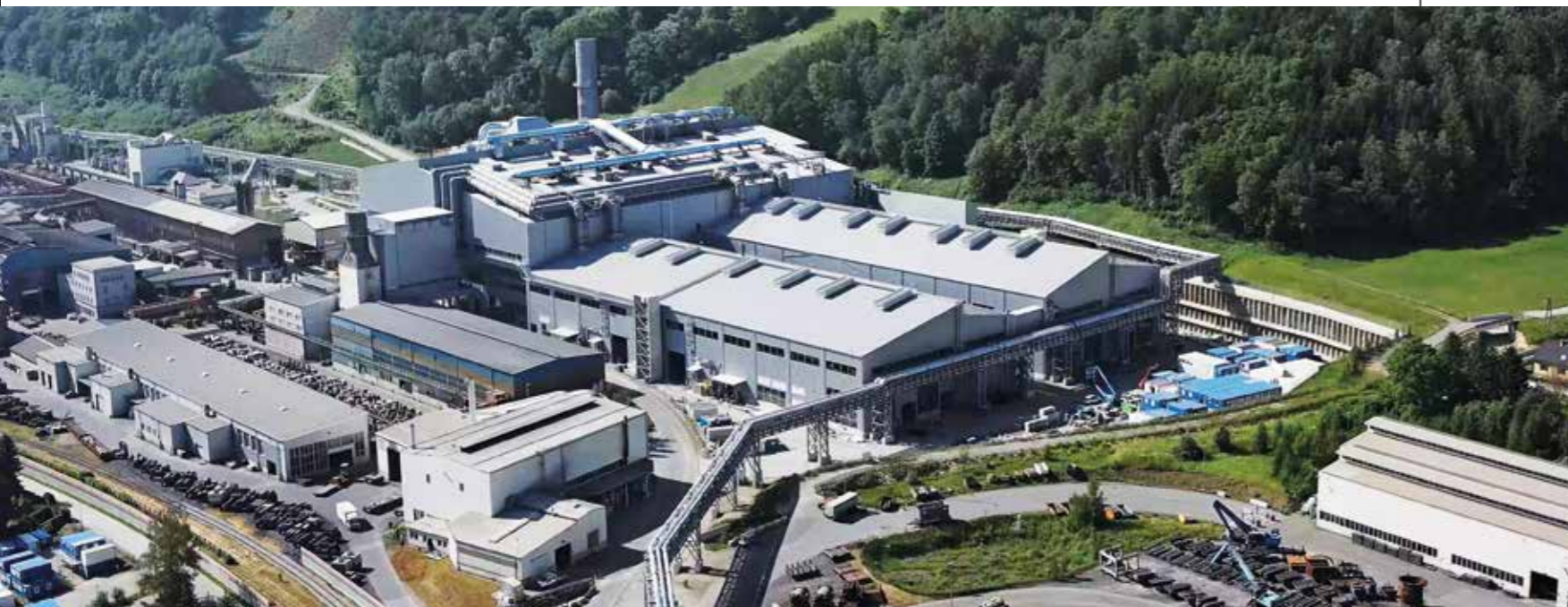
The new electric steel plant in Kapfenberg sets new standards in production quality, process reliability and environmental practice.
