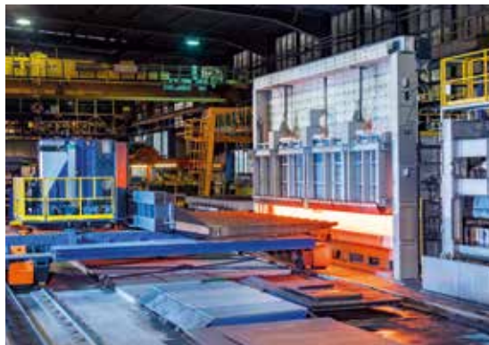
Heat treatment furnace
