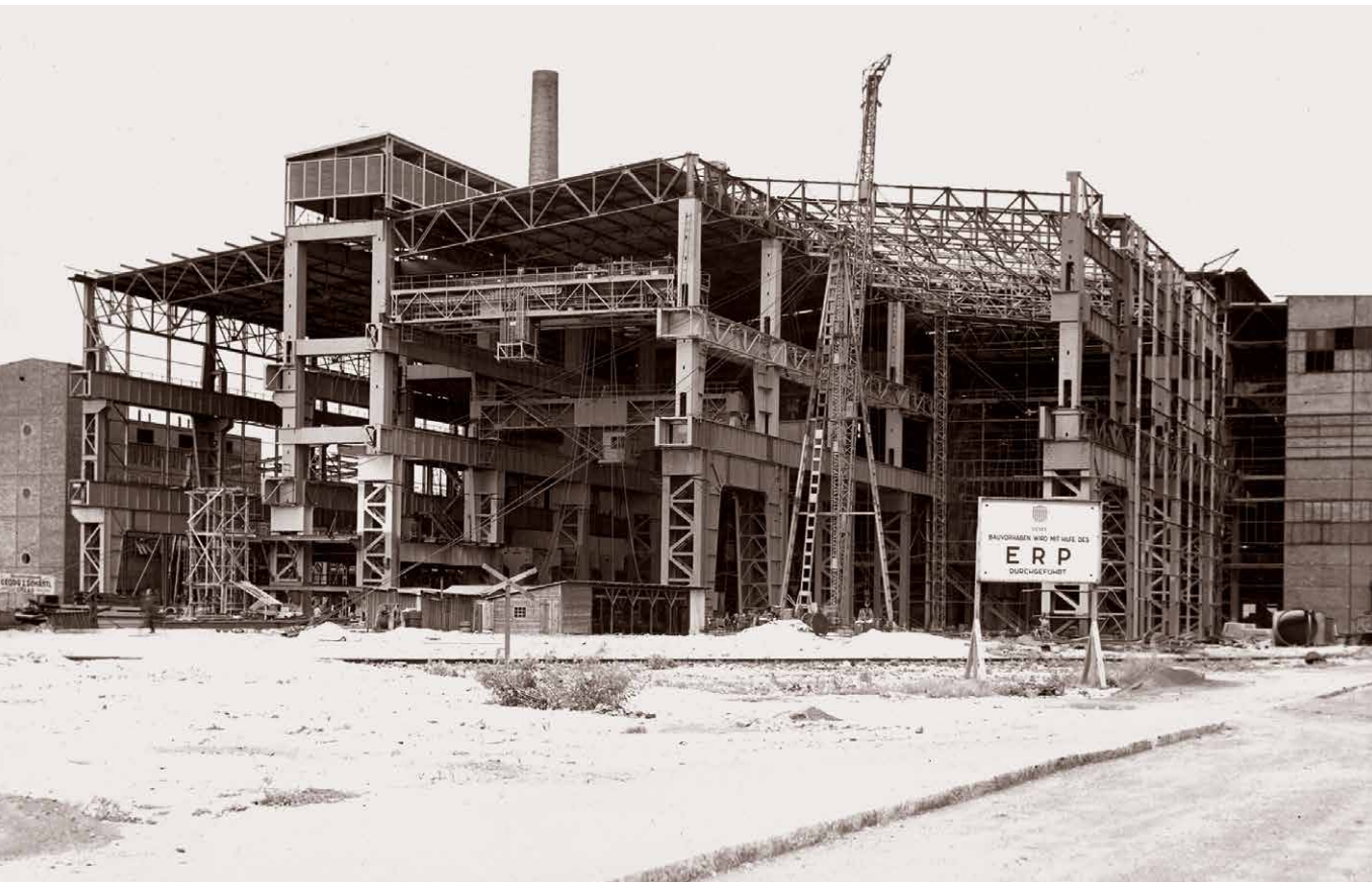
VÖEST LD Steelworks 1 under construction.
