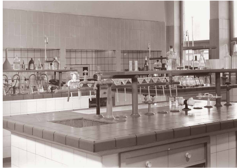
A steelworks laboratory in the 1950s.
